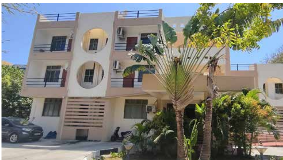
Repair and painting of Trainees' Hostel
