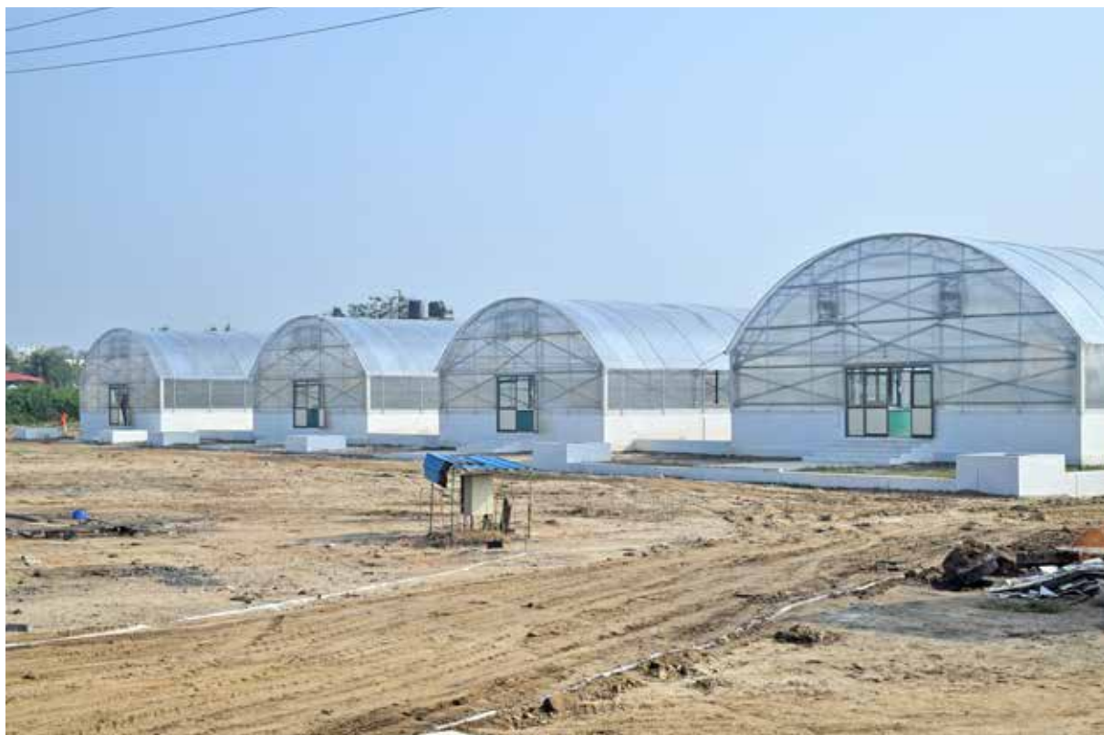
Construction of shrimp Nucleus breeding Centre
