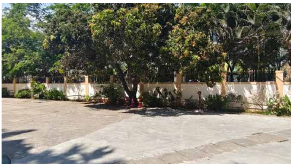
Repair and painting of compound wall
