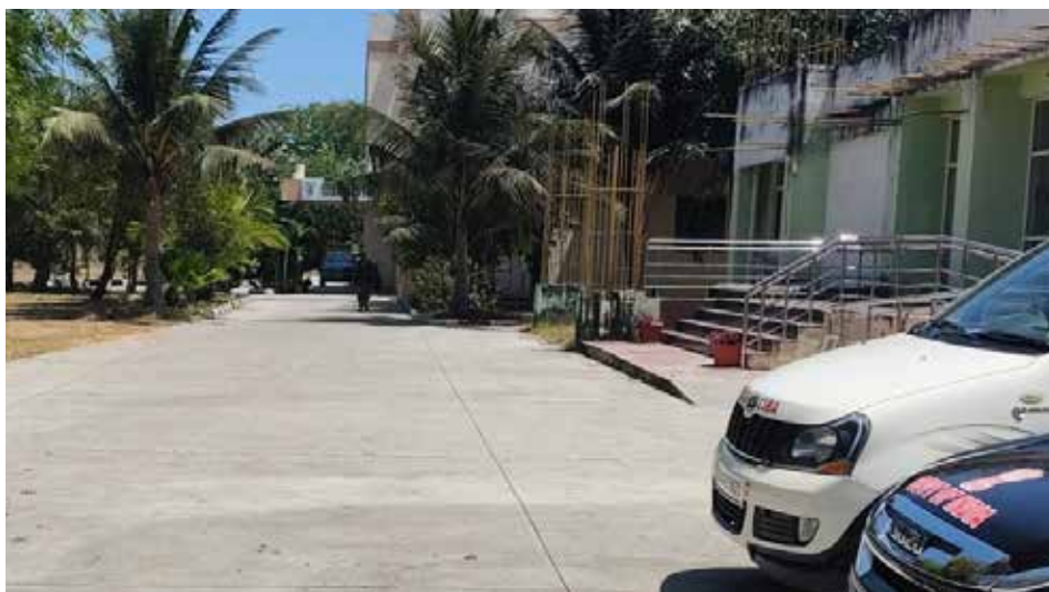
Repair of internal roads
