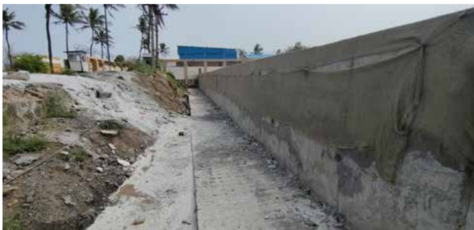
Restored wall at hatchery entrance gate
