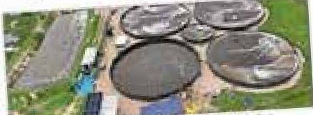
PROJECT: Aerial view of CIBA's new shrimp farming system.
