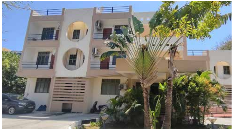
Repair and painting of Trainees' Hostel
