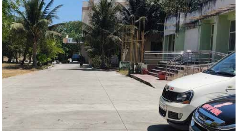
Repair of internal roads
