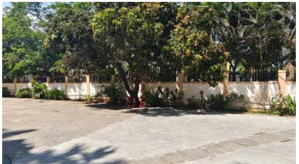
Repair and painting of compound wall
