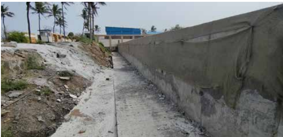
Restored wall at hatchery entrance gate
